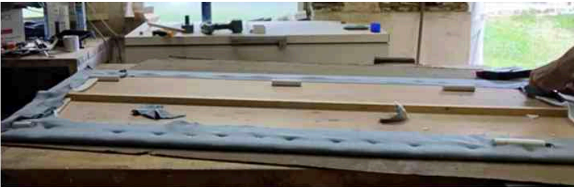
Staple fabric (evenly) and cut off excess.
